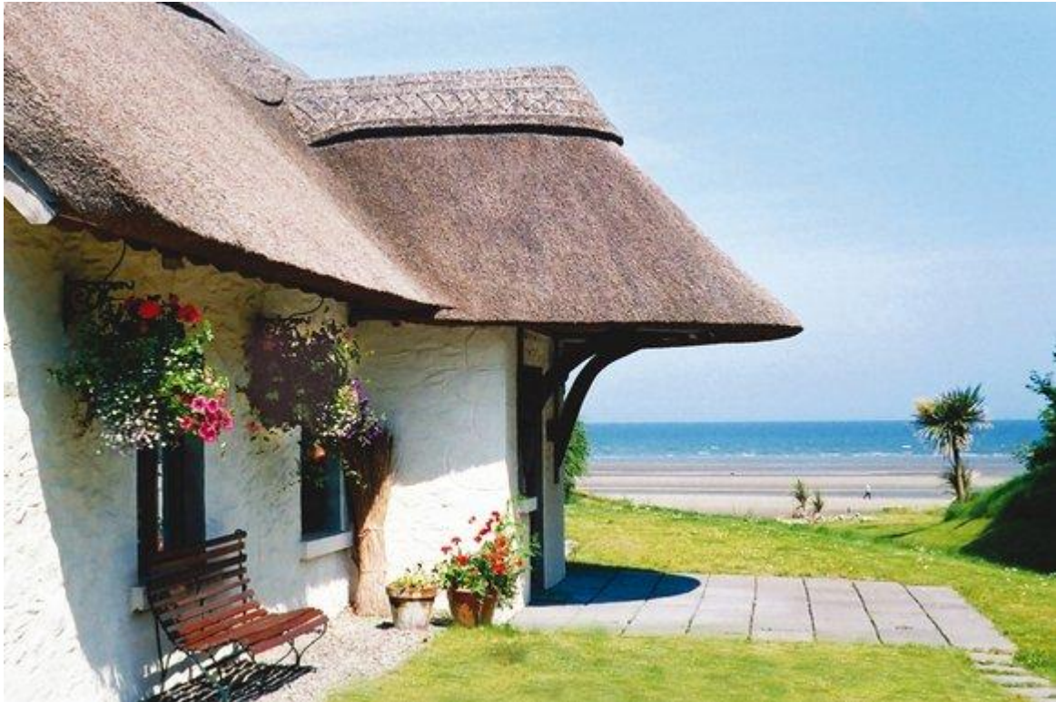
48. Thatchers Rest Cottage, The Cottages Bettystown, Ireland
